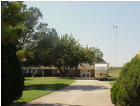
Figure 7: Wind turbines tend to blend into the background with distance. Lattice towers blend more quickly than monopoles. This 10 kW turbine system is located approximately 250 feet behind the house on a 100-foot guyed-lattice tower.
