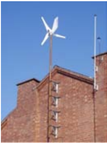
Figure 4: Building-mounted wind turbine.
